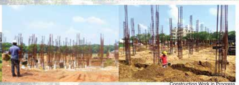
Construction Work in Progress
