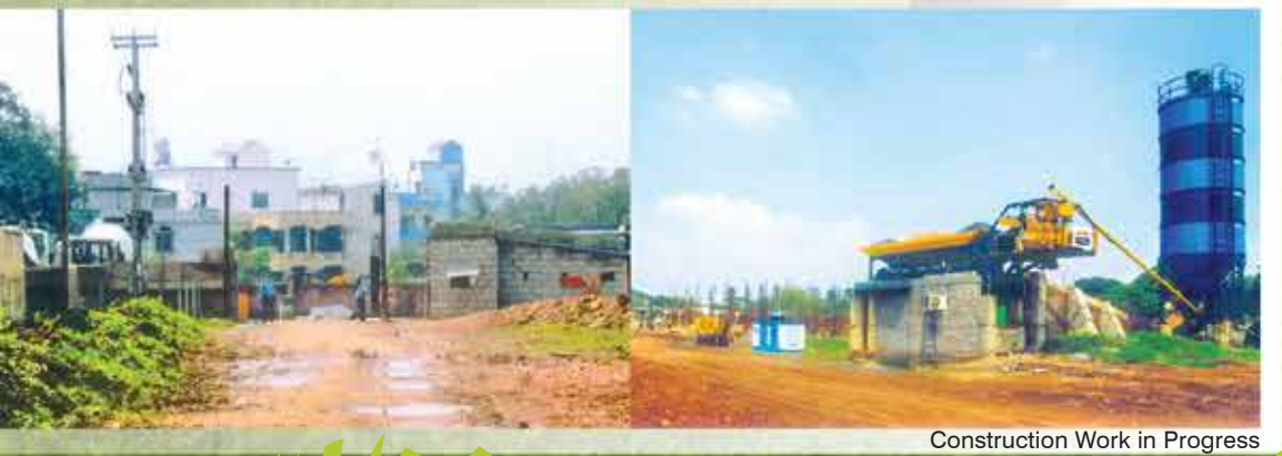
Construction Work in Progress
