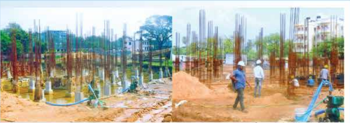
Construction Work in Progress
